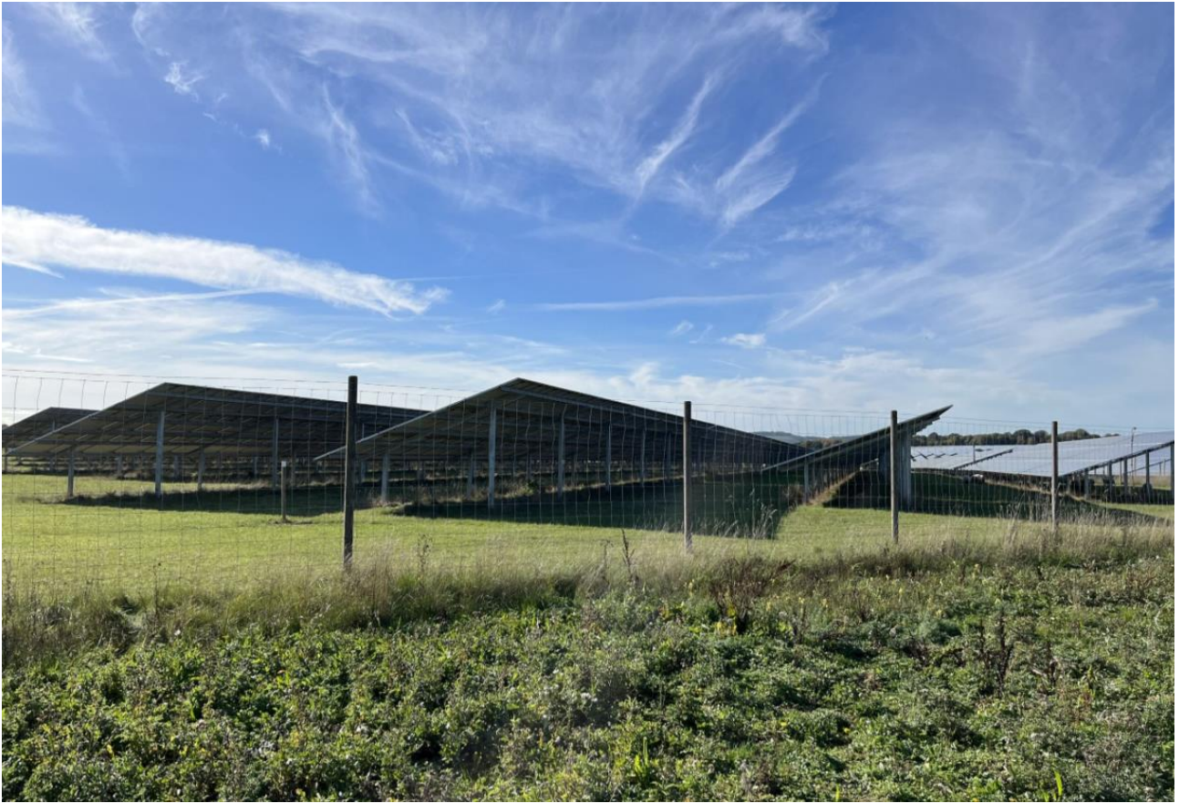
Plate 2-1: South-facing fixed tilt modules, finished array
