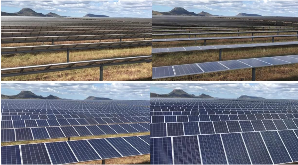
Plate 2-2: East-west single axis tracker system, finished array
